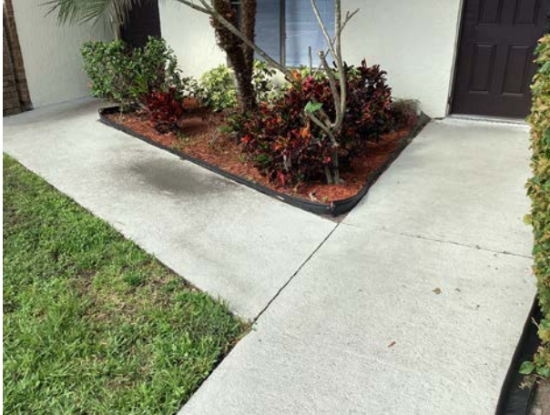
Concrete sidewalk at unit entrances
