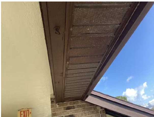
Aluminum soffit
