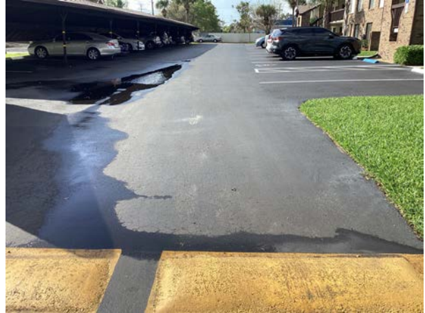
Asphalt pavement street overview
