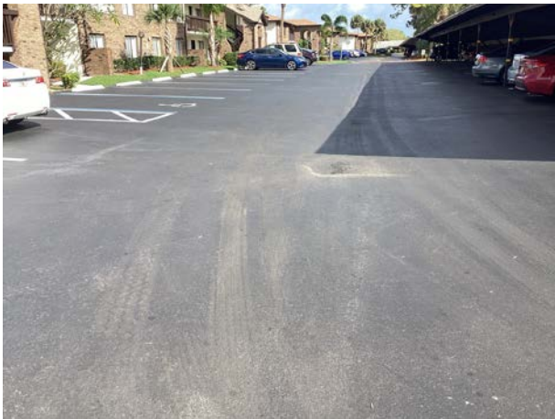
Asphalt pavement street overview
