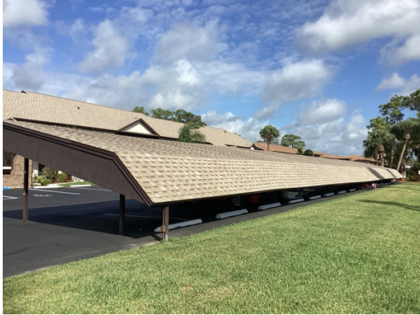
Car port roof
