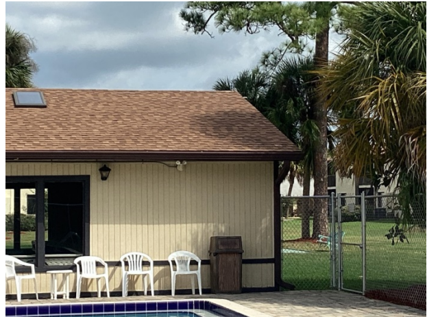
Pool house asphalt shingle roof
