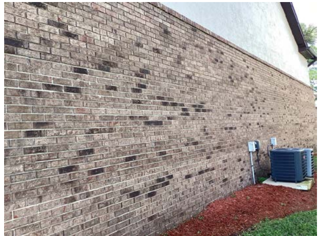
Masonry walls overview
