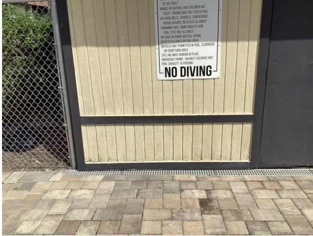
Wood siding at pool house
