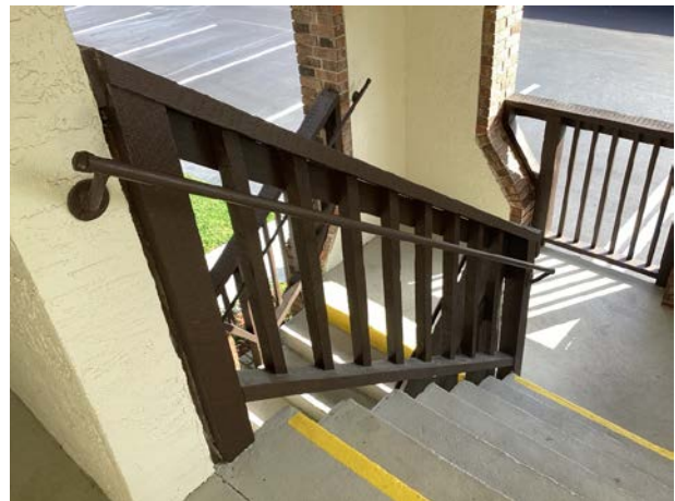
Wood railing at staircase
