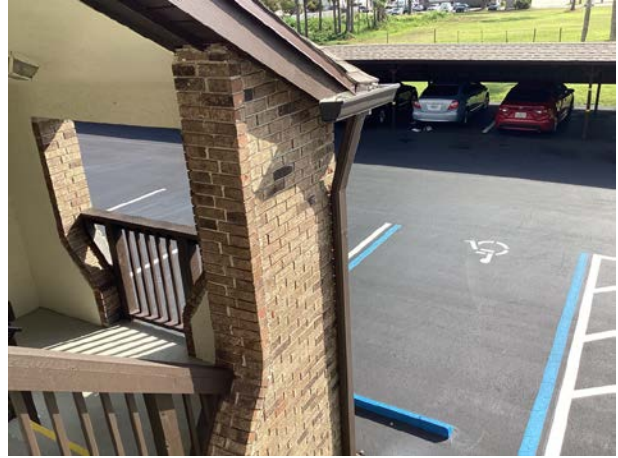
Gutter and downspout
