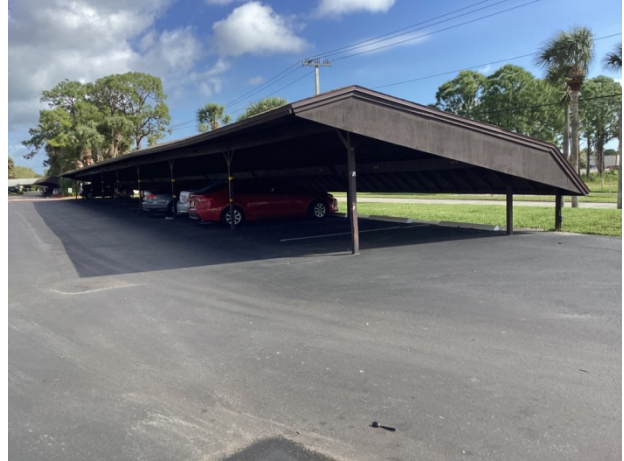
Car port structure
