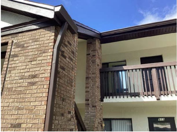
Aluminum gutters and downspouts
