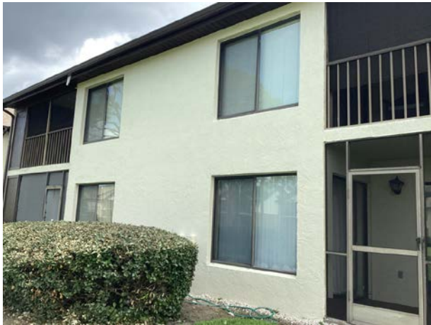
Stucco wall finishes
