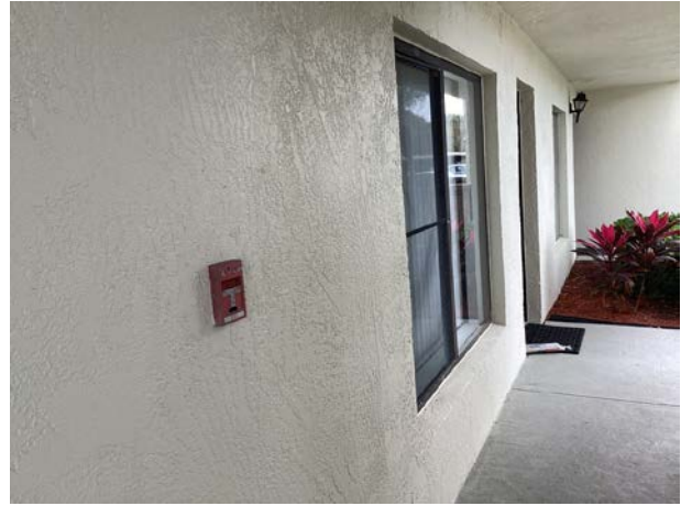
Stucco wall finishes
