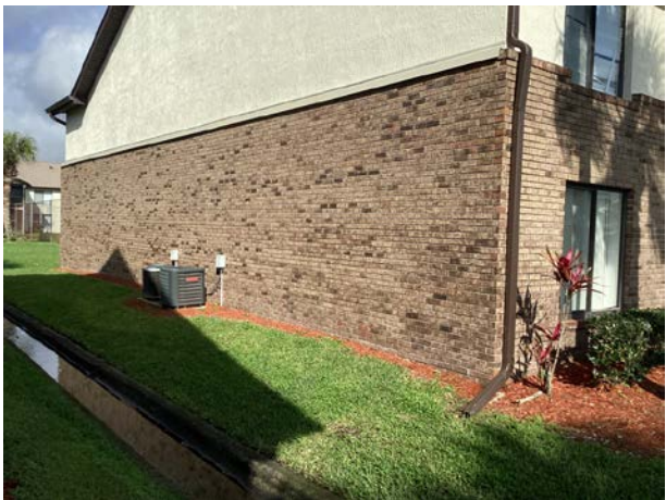
Masonry walls overview
