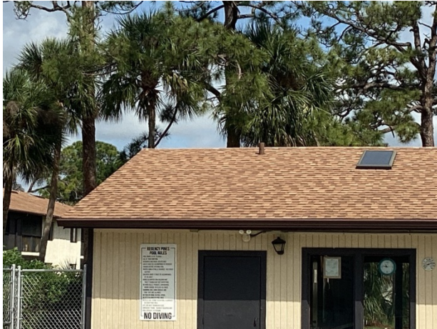
Pool house asphalt shingle roof
