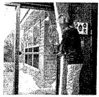
Since they slide horizontally, it is important to have a blocking device in place to prevent sliding the door fully open from the outside. You can do this by inserting a wooden dowel or stick into the track thus preventing or limiting movement. There are also metal fold-down blocking devices called "Charlie bars" and various track-blockers that can be screwed down.
